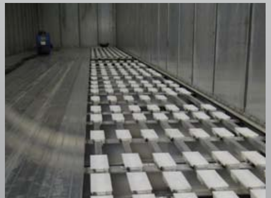
Floor with continuous lateral reinforcement
